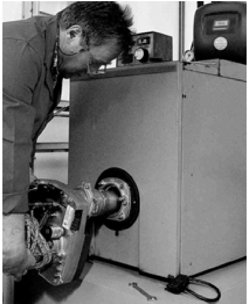
Abb. 11: Brenner-Kessel-Montage II
